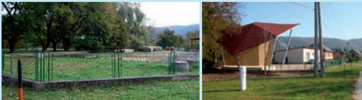
Hrušov: Public space before and after reconstruction
