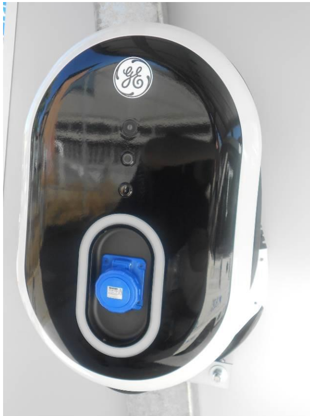
GE Wattstation wall mount
