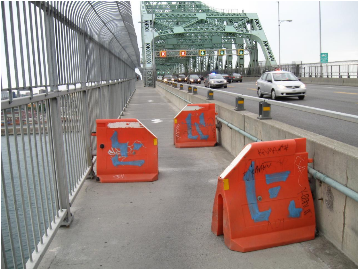
Figure. Bicycle traffic calming on downhill grade on bridge in Montreal, Quebec, Canada. (Photo Jason Meggs)
