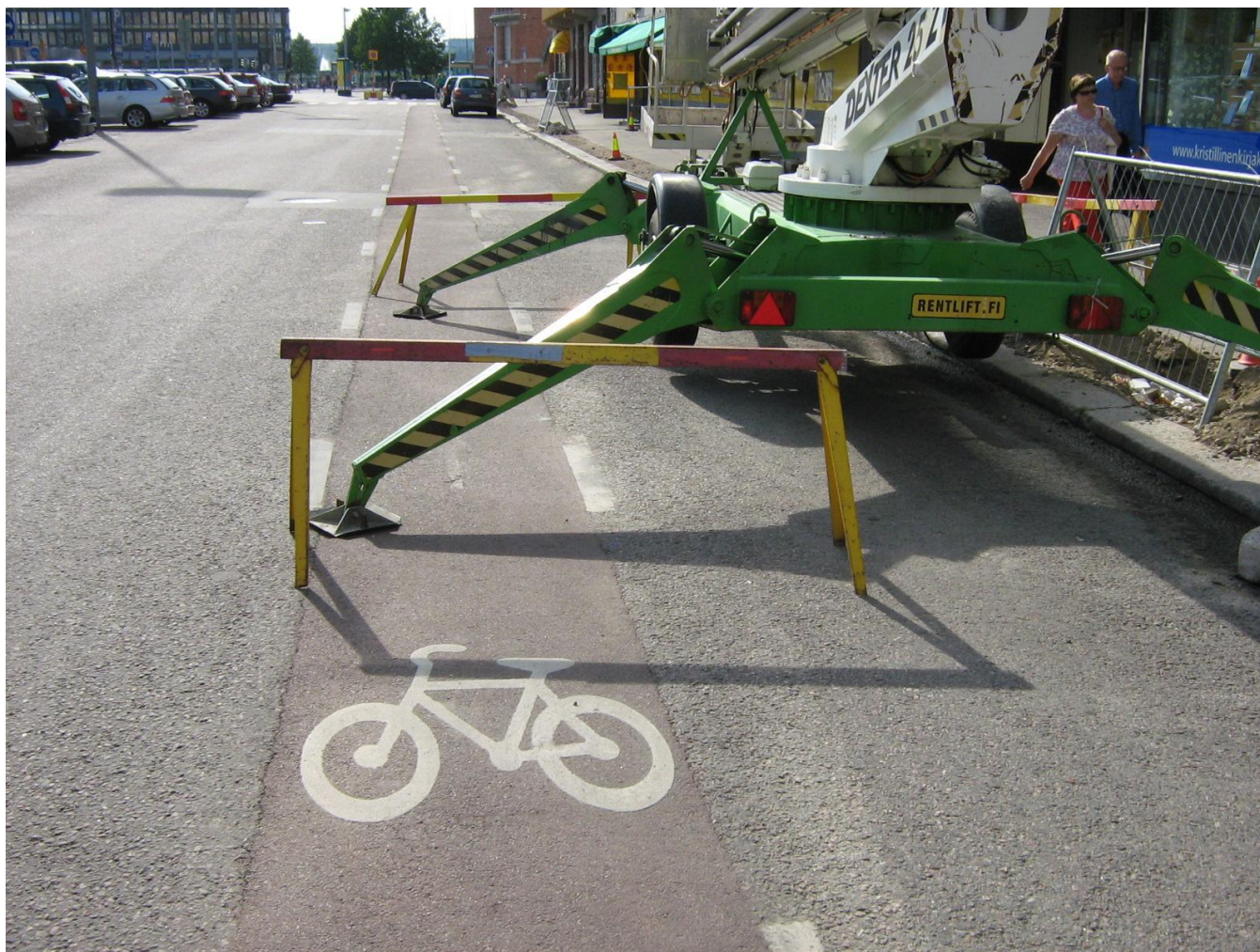
Figure. Construction often interferes with cycling. Photo Jason Meggs
