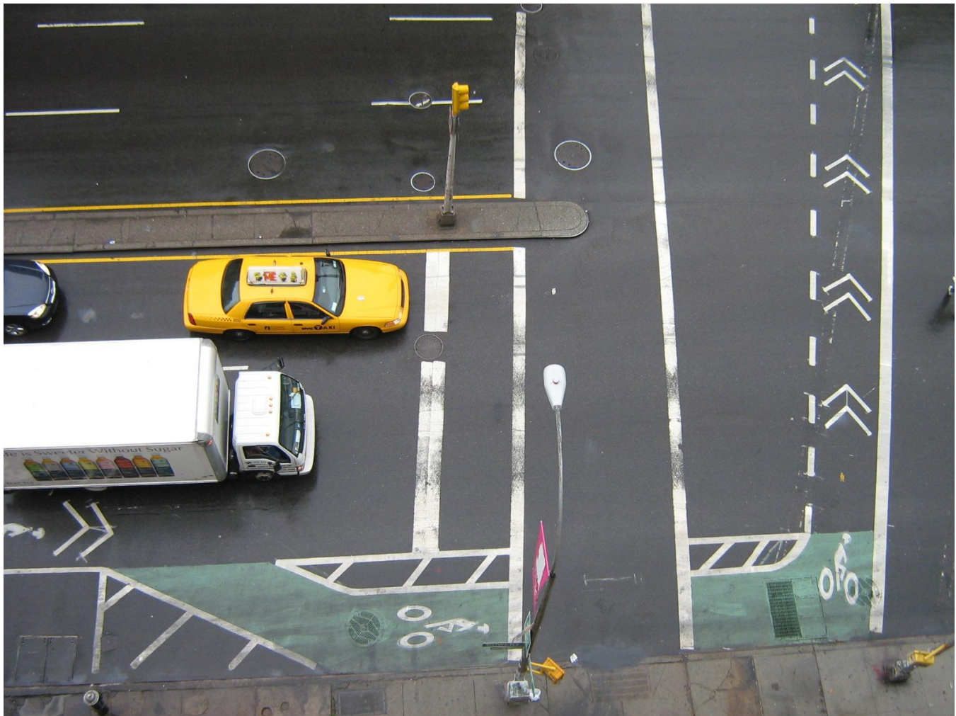
Figure. An innovation in New York City helping cyclists turn left across a dangerous intersection with heavy truck traffic. Prince and Bowery, NYC. (Jason Meggs)
