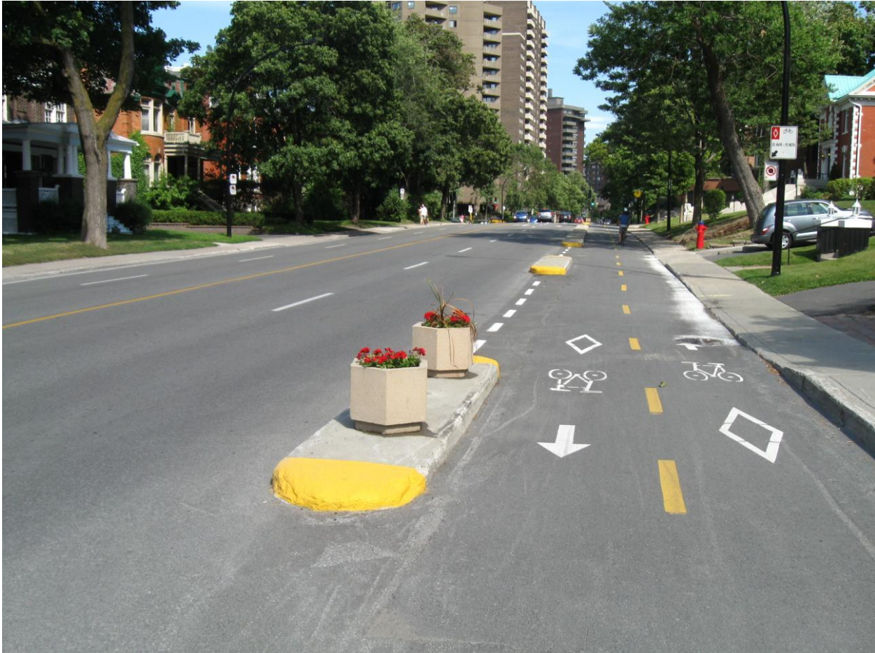
Figure: A relatively inexpensive and quick conversion of existing road space to include a bike path in Montreal, Canada. (Photo, Jason Meggs).
